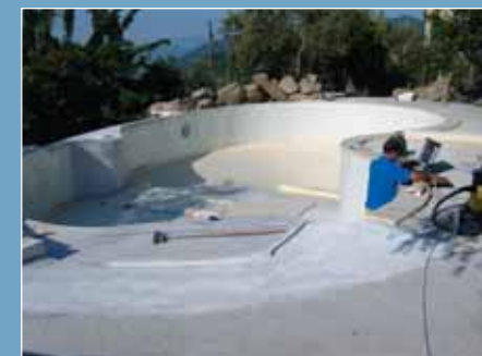
> Applying the PVC lining
