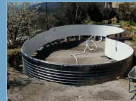
> Assembly of the structure
