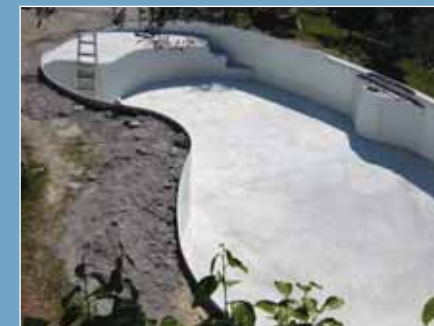
> Pouring the concrete floor, installation of accessories and filter system
