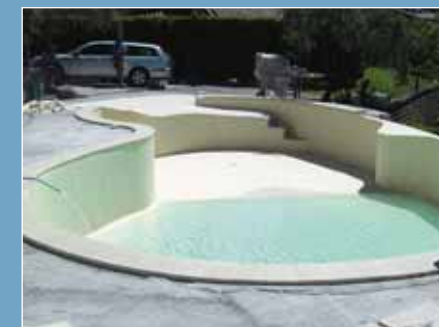
> Filling the pool with water
